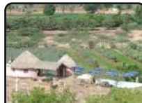
WATER PUMP STRUCTURE
