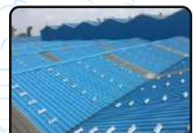
TIN SHADE STRUCTURE
